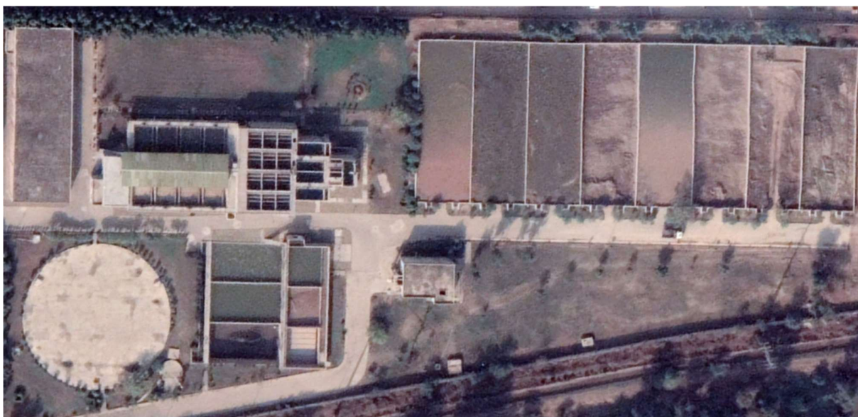
Figure 6: Satellite Image of 5 MGD Extension to 10 MGD WTP
